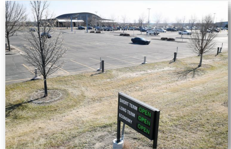
COVID-19 initially led to significant impacts to passenger demand and greatly impacted local revenue streams for the airports.
