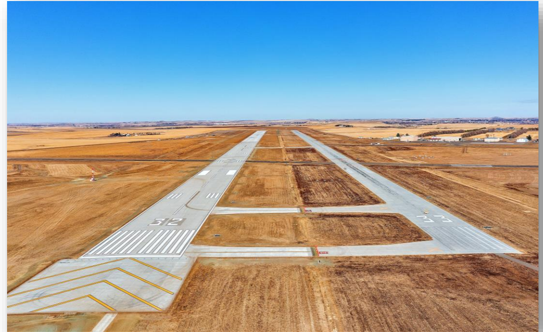
Dickinson Airport Primary Runway Construction (2022)
