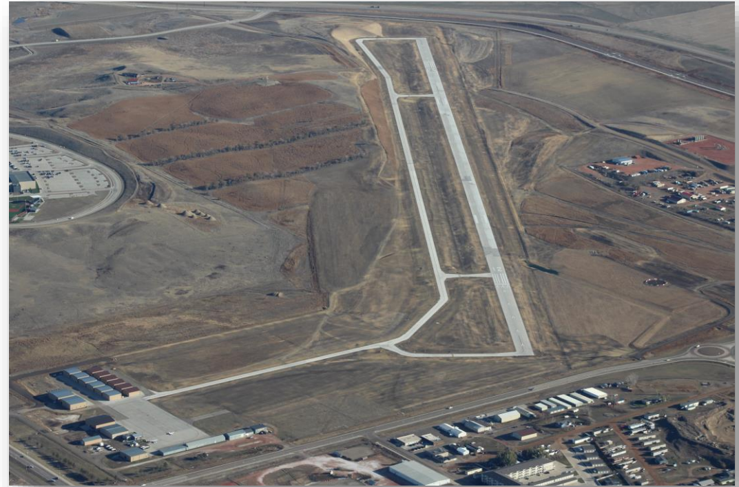
Watford City Airport Runway Reconstruction & Extension (2021)
