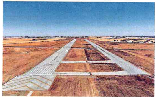
Dickinson Airport Primary Runway Construction (2022)
