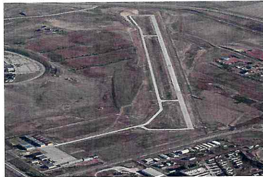
Watford City Airport Runway Reconstruction & Extension (2021)
