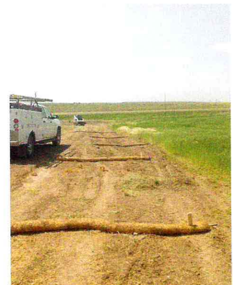
Same site after reclamation
