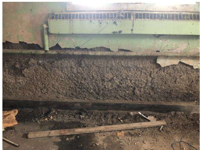
Image 7: Damaged Foundation Wall
