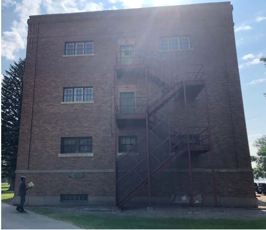
Image 1C: Building 16 East (West Elevation)
