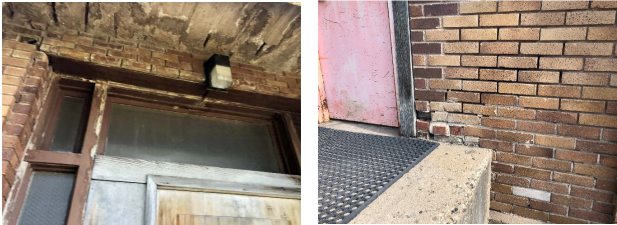
Image 3: North Entrance (Left) South Entrance (Right)
