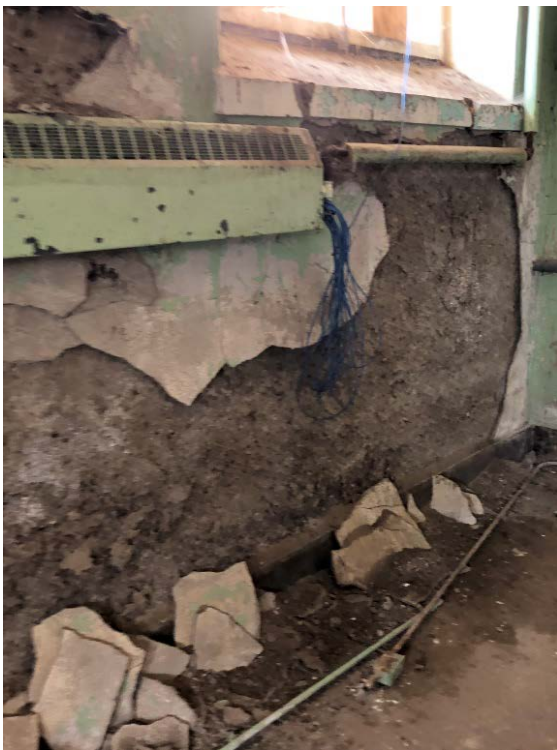
Image 7: Damaged Foundation Wall
