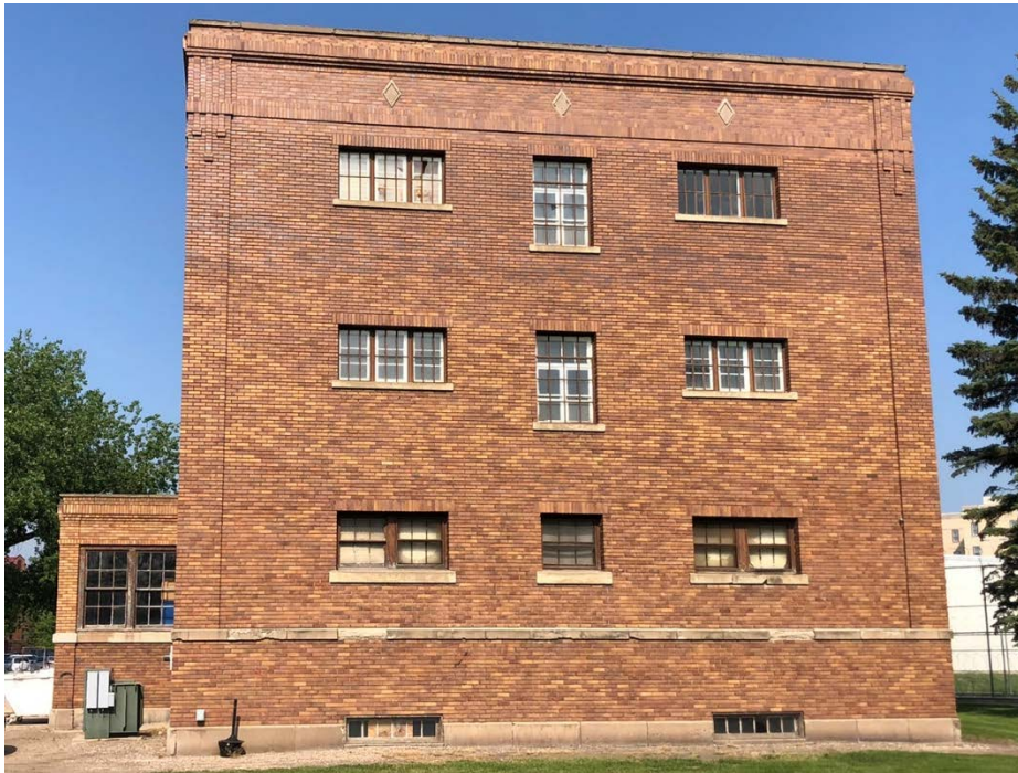
Image 1D: Building 16 East (East Elevation)
